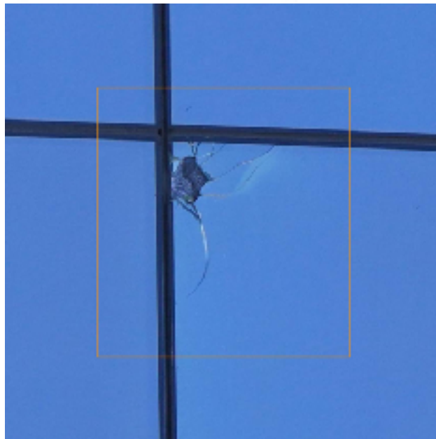
Cracked Glazing
