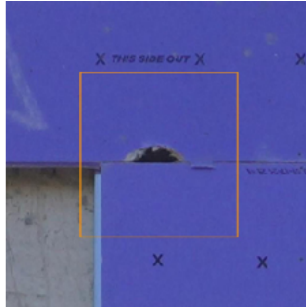
Damaged sheathing
