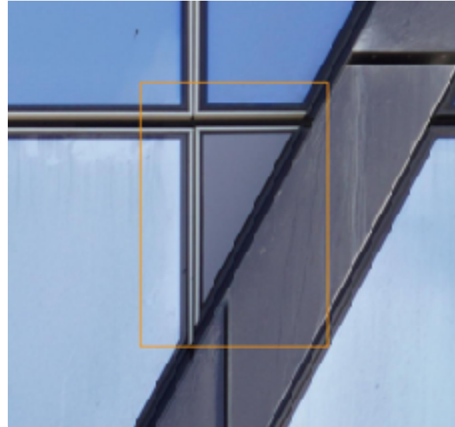
Wrong glazing type installed
